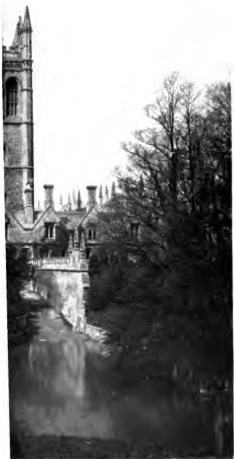
GDALLEN TOWER Oxford
